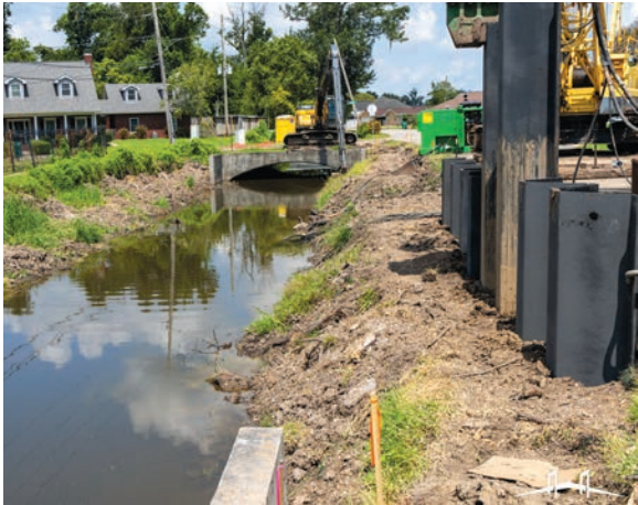
Construction continues on the parish's $1.5 million Phase 1B Primrose Canal project.
