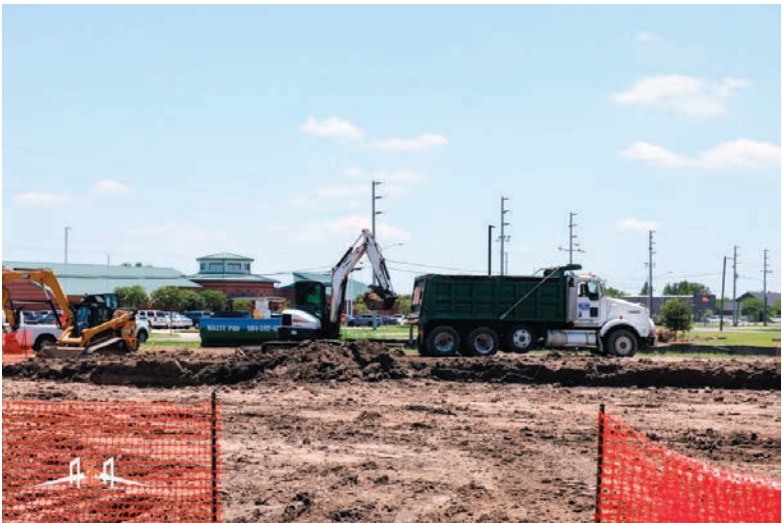
The parish hopes to complete construction of sand volleyball courts near the Edward A. Dufresne Center by September. The $660,000 project began in May.
