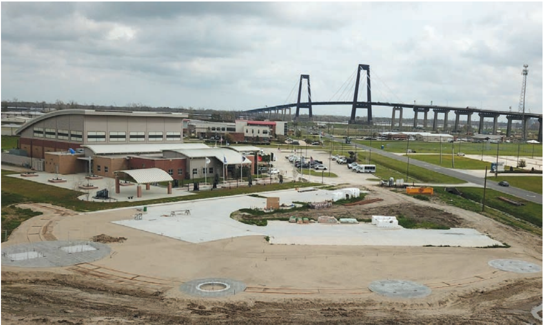
Work on the West Bank Spray Park is nearing 75 percent completion.
