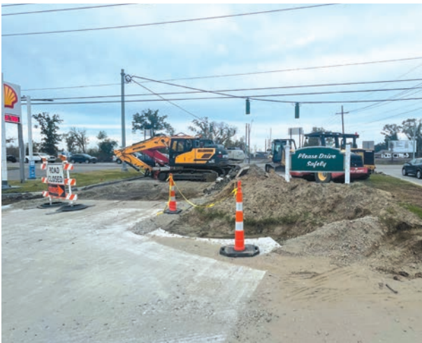
Ongoing work where Lakewood Drive meets Highway 90, one of the last portions left before the reconstruction project is complete.
