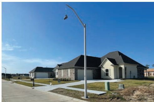
Recently constructed homes await buyers in the Heather Oaks subdivision of Luling.
