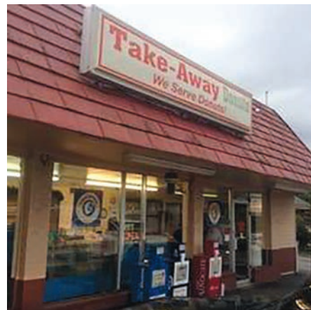
Exterior view of Takeaway Donuts prior to sustaining storm damage in 2021.
