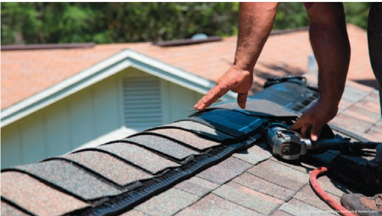
Roofer nailing a ridge cap on an asphalt shingle roof.
