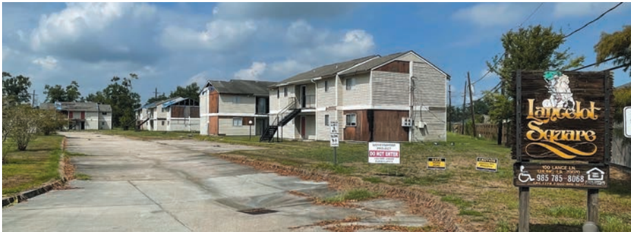
The Lancelot Square Apartments complex in Luling prior to the start of demolition work in late August.
