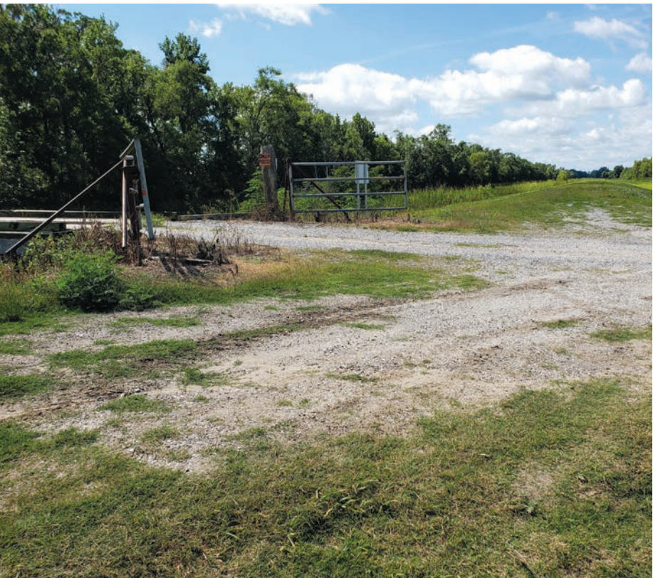
Gated area and levee section part of the upcoming Sunset Levee lift project, which will add additional storm and flood protection to the Bayou Gauche area.
