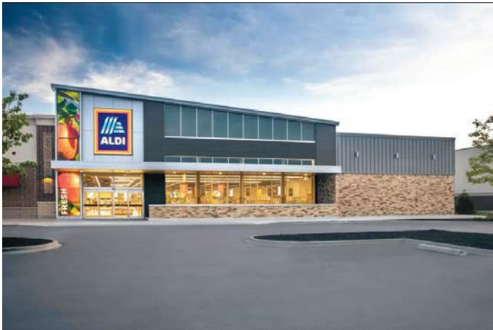
ALDI corporate images showing typical ALDI grocery store exterior and interior layout designs.
