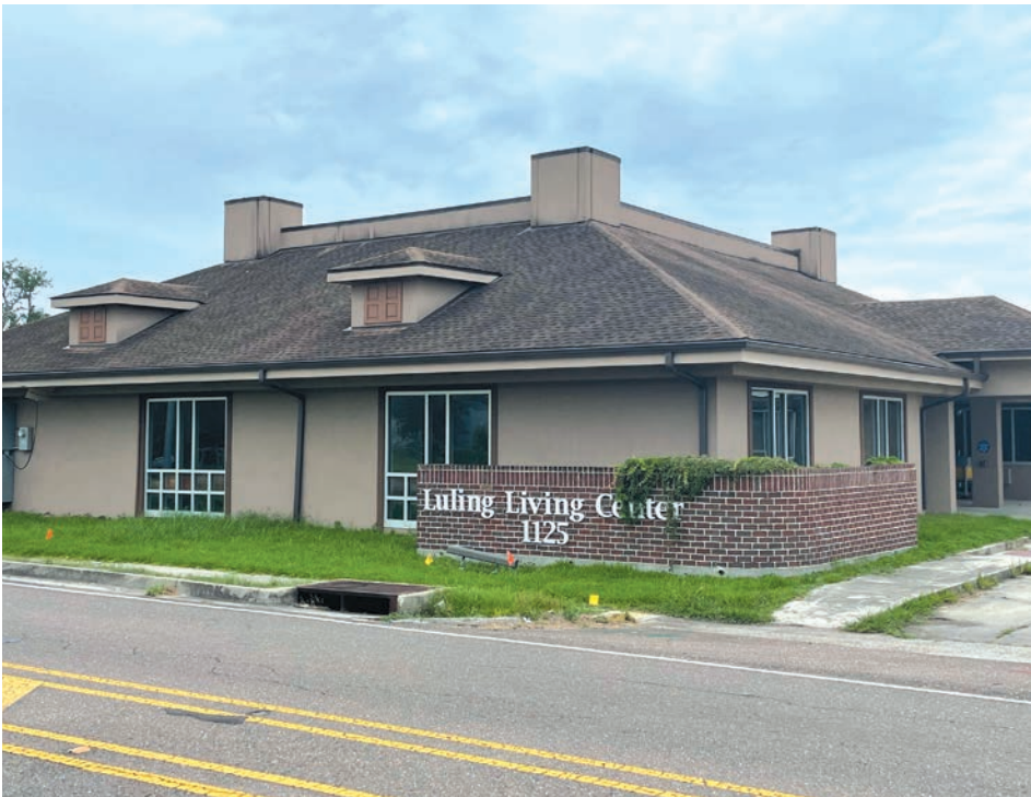
Exterior photo of Luling Living Center on Paul Maillard Road, which is set to receive a new pitched metal roof later this month.
