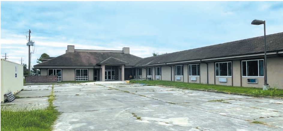
The currently vacant Luling Living Center facility awaits the start of staged gut and rehab work later this year, with current projected reopening set for August 2024.
