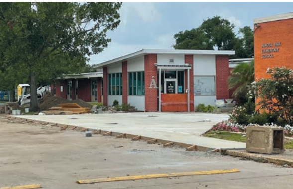
Canopy, concrete and related renovation work currently underway at Mimosa Park Elementary School on Birch Street in Luling.
