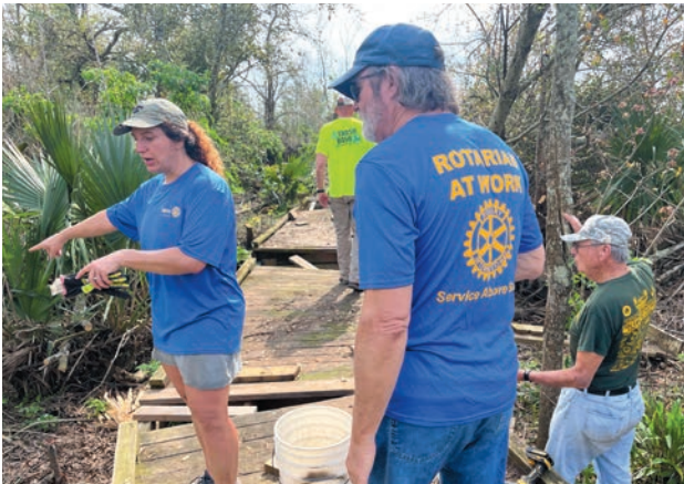
Volunteers coordinate cleanup efforts and boardwalk repair work at Wetland Watchers Park in Norco.
