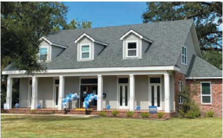
Exterior photo of CAS of Destrehan’s offices located at 13726 River Road.
