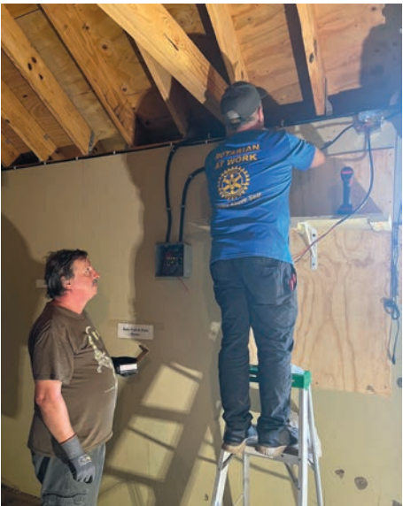
Rotary Club volunteers work to shore up and repair the Wetland Watchers Park’s storage building.
