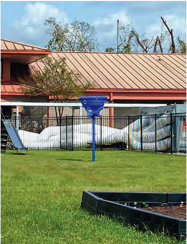
Roof replacement at New Sarpy Elementary is one of the hurricane-related projects left to complete.
