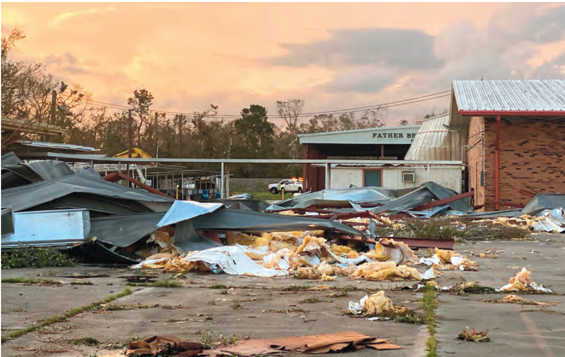
The grounds and buildings of St. Gertrude the Great Catholic Church were severely damaged by Hurricane Ida.
