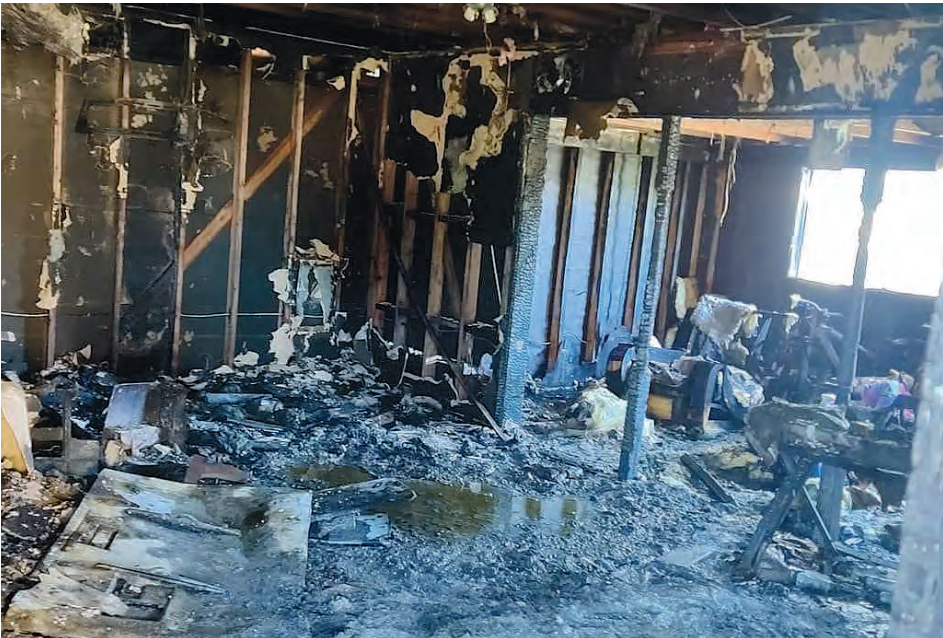
(Top) The family’s home was completely destroyed by an electrical fire.
