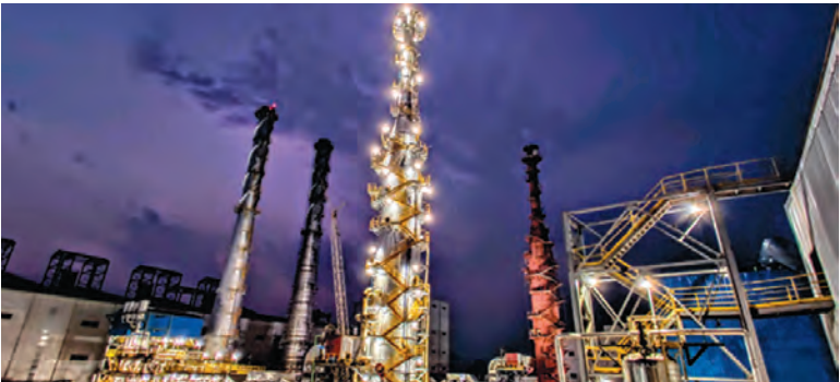
Flue-gas desulfurization systems installed at four of Rain Carbon’s plants in the United States and India remove as much as 98 percent of the sulfur dioxide from its emissions.
