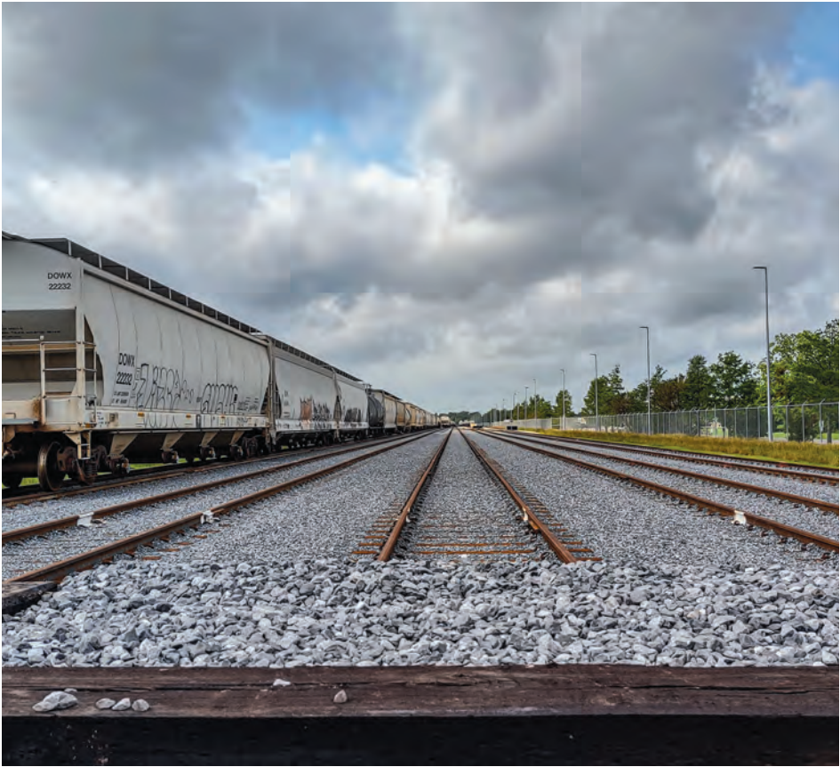
The Port recently announced the completion of a six-track rail yard storage project in St. Charles Parish.
