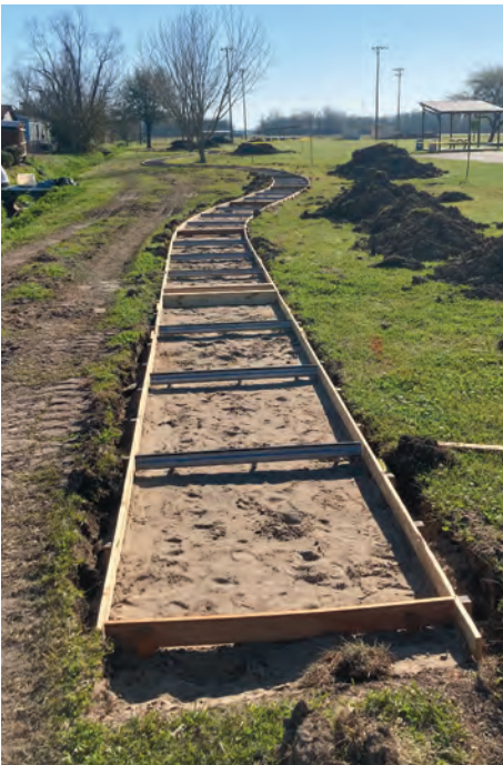
Construction on a walking path in Killona is also underway.
