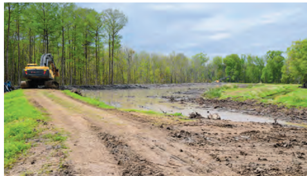
Parish employees work on the West Bank portion of the levee.
