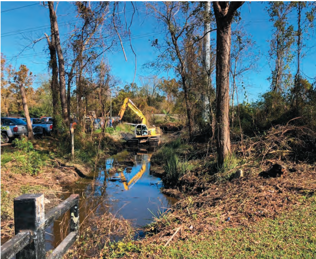
Extensive culvert and drainage work in Destrehan took place in 2021 and should be completed by the end of January.
