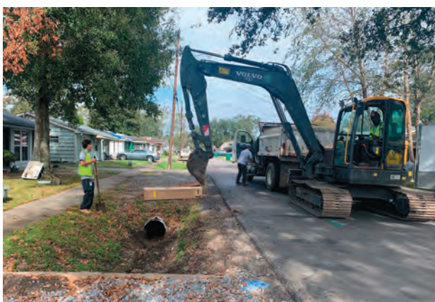
Drainage work takes place on Marino Drive in Norco.
