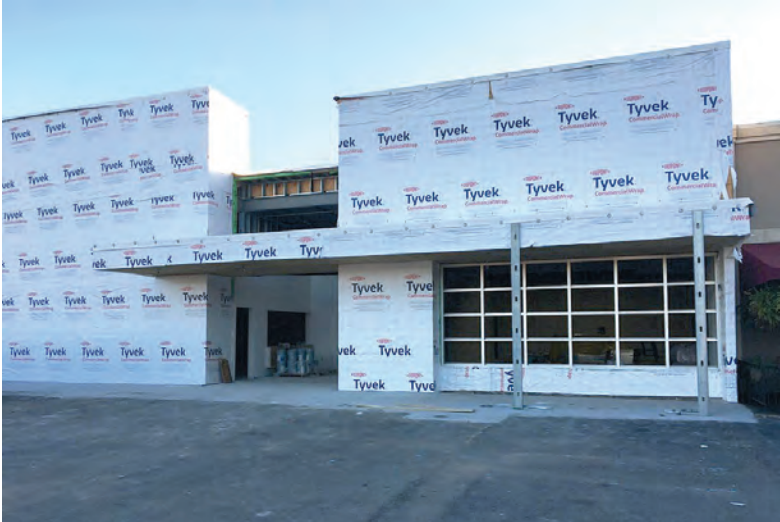
Construction work is progressing on the River Parishes Community College - United Way campus.
