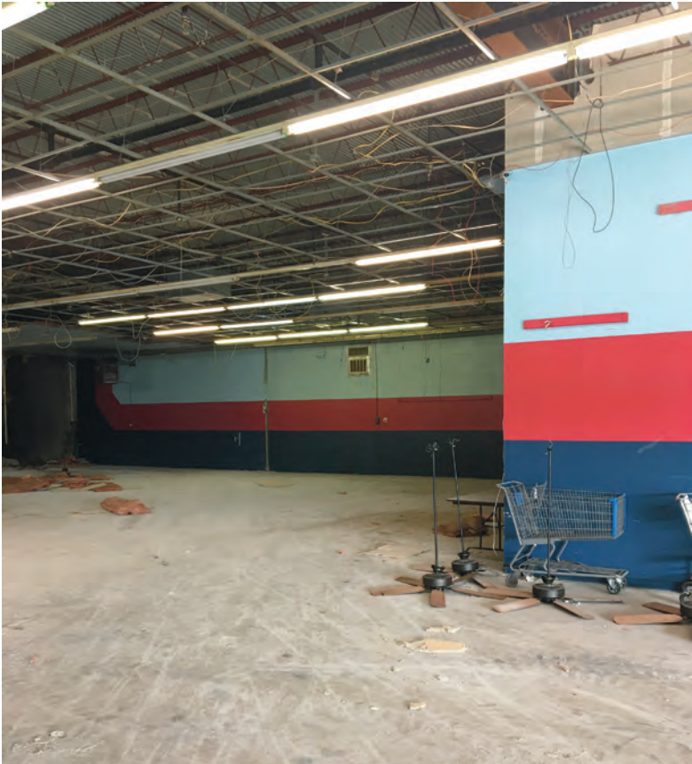
Pictures showing ongoing construction that began in July.
