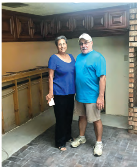
Terry and Vicki Caillouet stand inside their flood damaged home.
