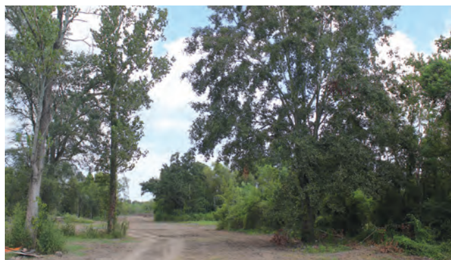
Site work previously underway on now canceled Saints Place Subdivision in Destrehan.
