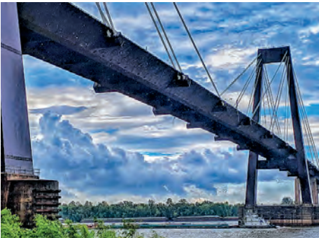
Hale Boggs Memorial Bridge in Luling.
