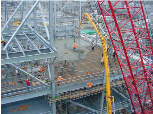
Expansion construction underway at the Bayer plant in Luling.
