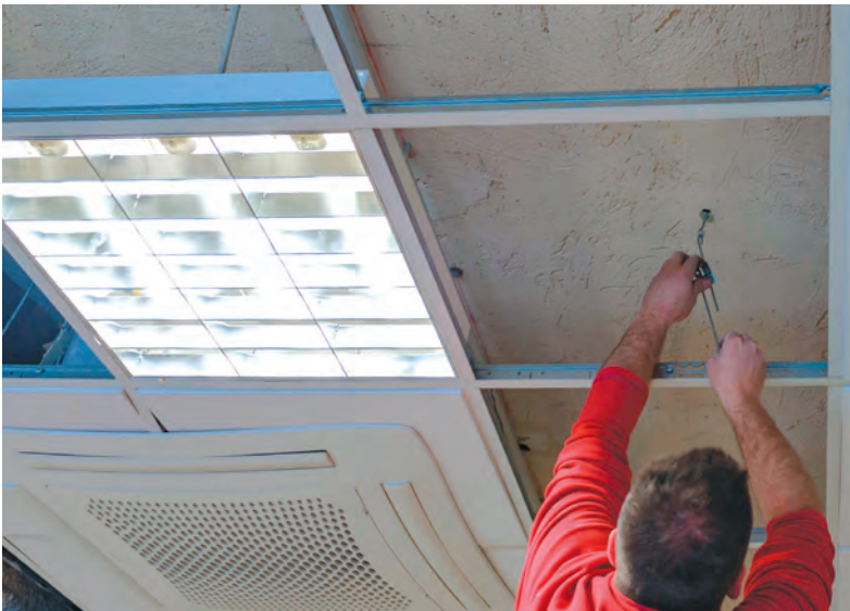
Repairs and renovations are underway at several school sites.
