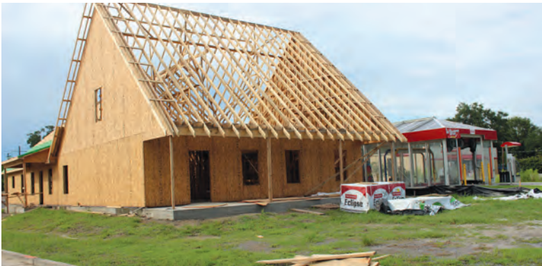
Construction underway for the new State Farm insurance office on U.S. Highway 90 in Boutte.
