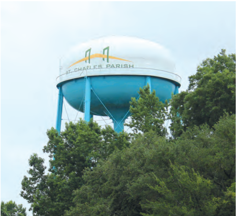
One of three water towers in St. Charles Parish set for demolition.
