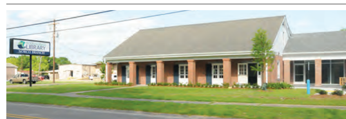
The new site of the parish's Norco library, which is set to open soon.
