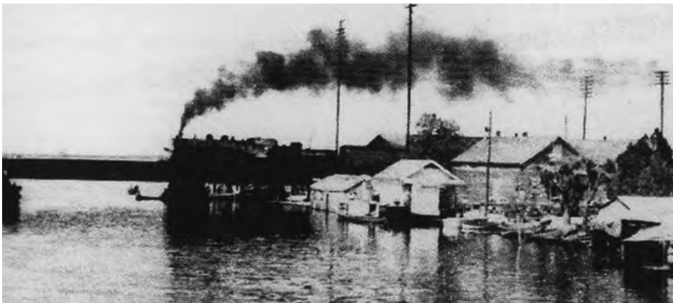
Train crossing over Bayou Des Allemands.
