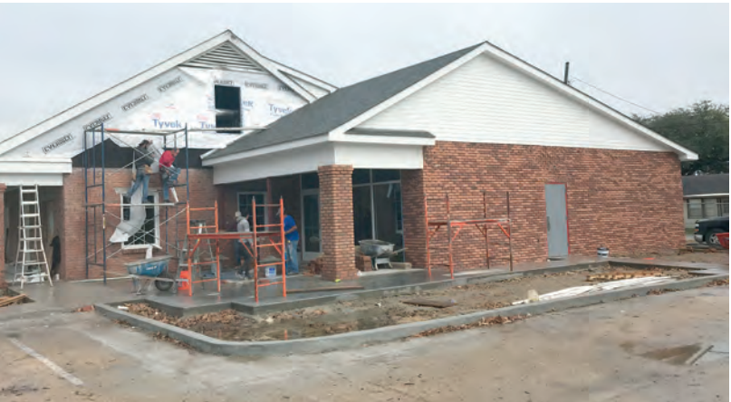
Exterior work underway on the new Norco Library.
